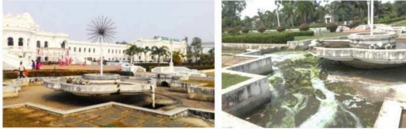
FIGURE 12 EXISTING CONDITION OF THE FRONT GARDEN
