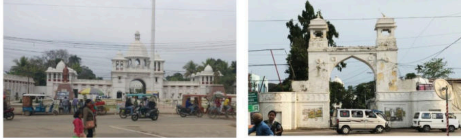
FIGURE 4 SOUTH GATE AND NORTH GATE STRUCTURES
