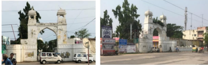
FIGURE 14 EXISTING CONDITION OF THE NORTH GATE
