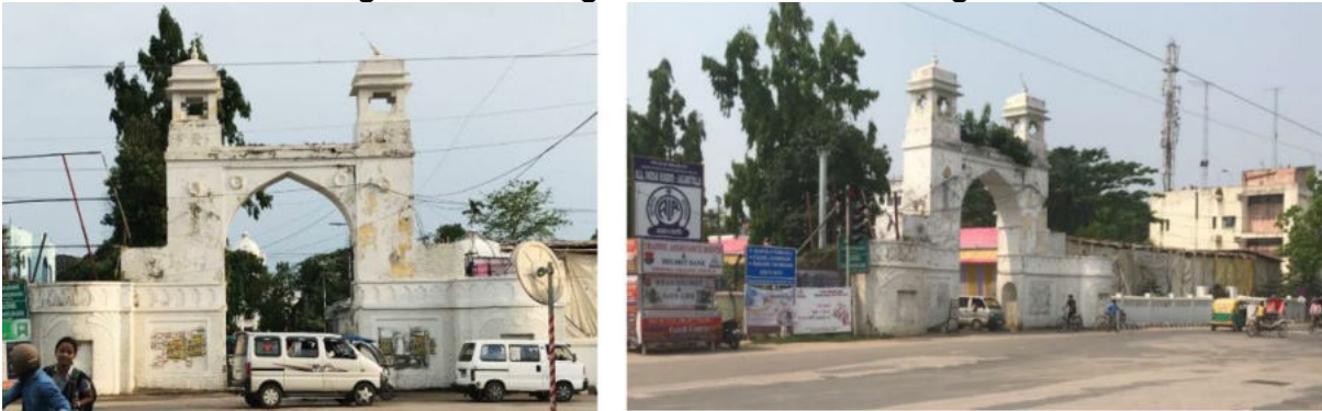
Figure 4: Existing condition of the north gate
