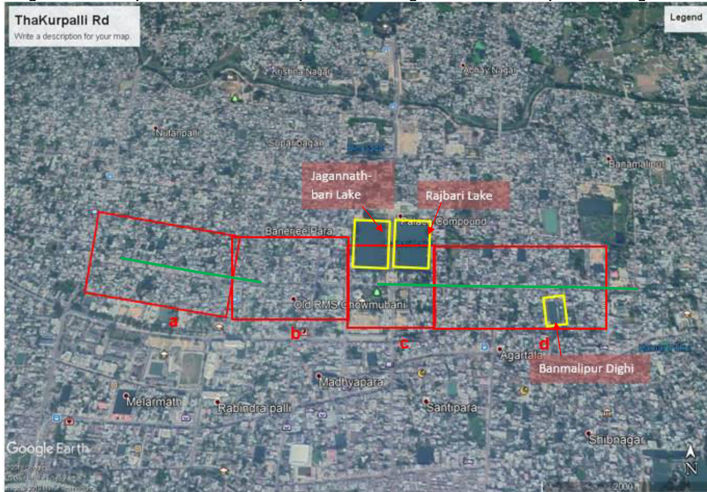
Figure 49: Thakurpalli Road Mixed Developed stretch along with sensitive receptors on Google Earth image
