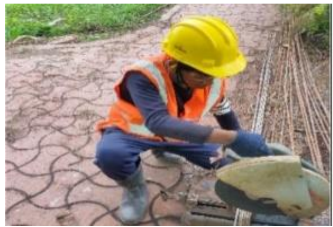
Use of hand gloves during cutting of steel rod at Ujjayanta Palace
