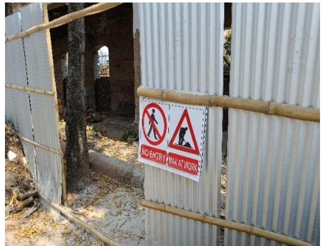
GI sheet – hard barricading at Astabal Area
