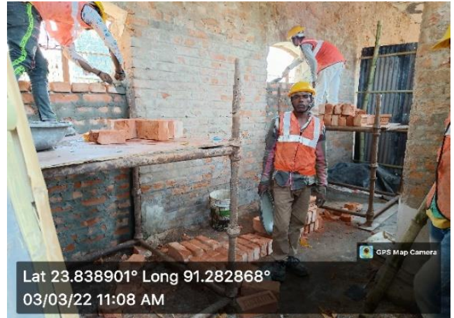
Work started at Astabal Area
