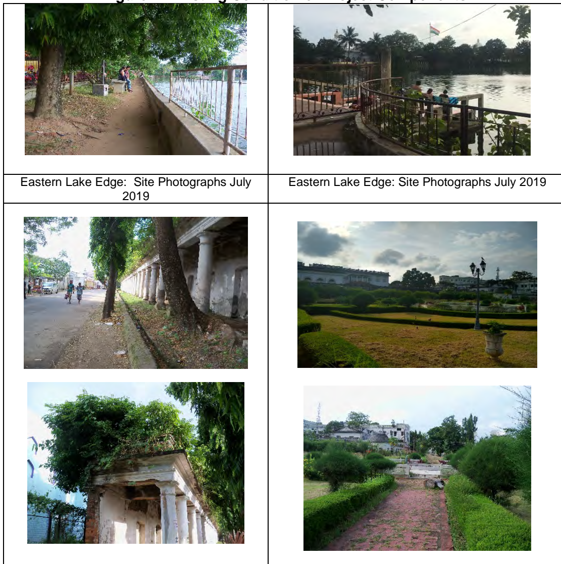
Figure 4: Existing Condition of Project Components
