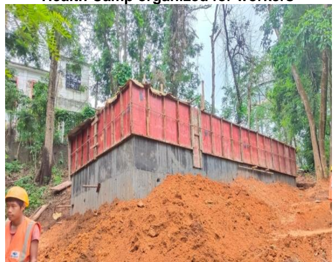
Machaan construction Work in Progress
