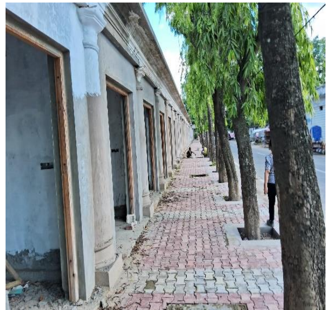
Astabal area finishing work under progress
