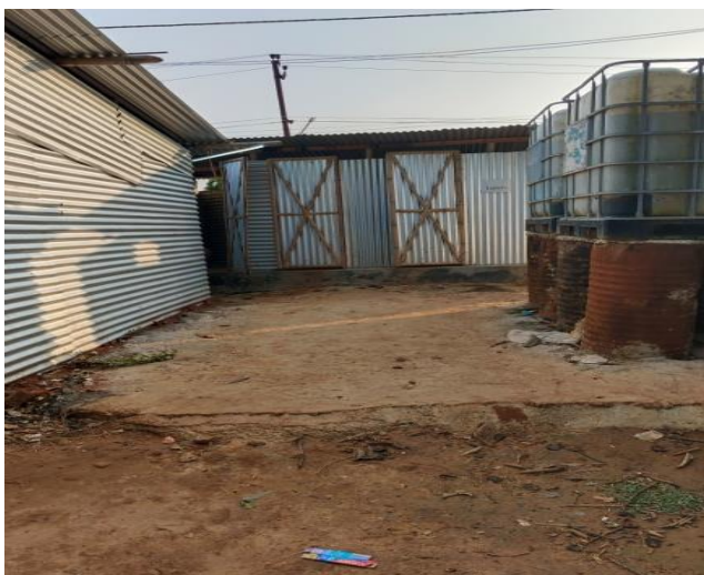
Toilet facility provided with septic tanks at labour camps
