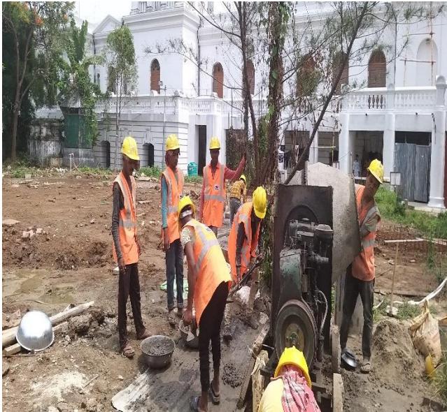
Use of PPEs by workers – noted
