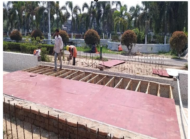
Shuttering work continued for bridge over the central channel
