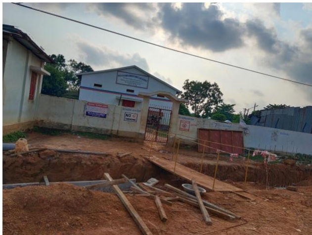
Temporary access provided for the residents
