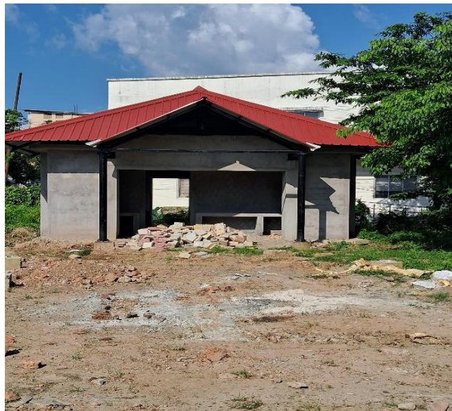
Food court 1 finishing work in progress
