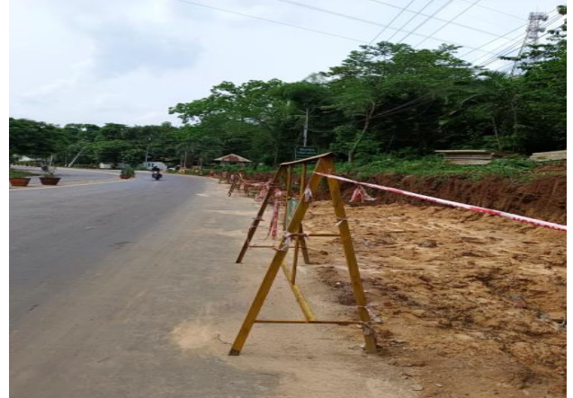
Work continued at VIP Road.
