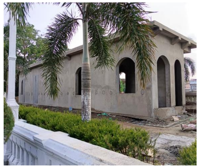
Plastering work for control room almost done at front garden
