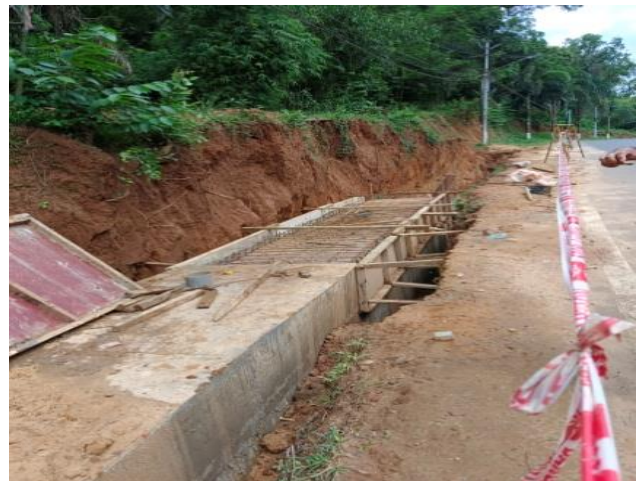
Work at VIP Road just started
