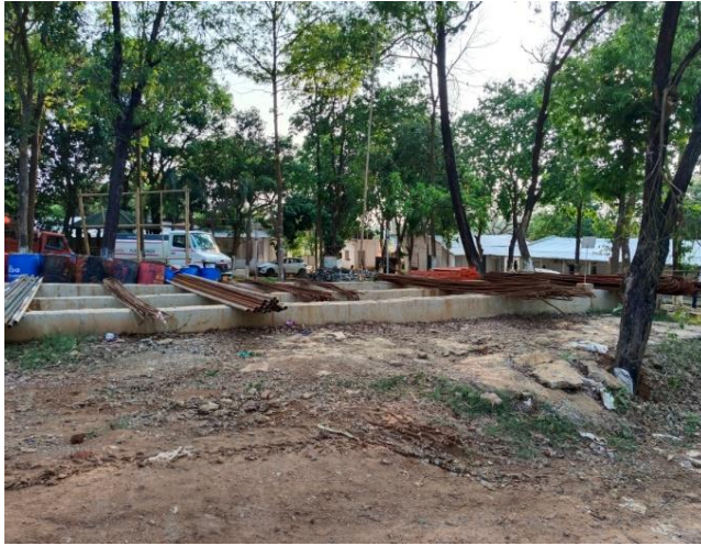
Proper material storage
