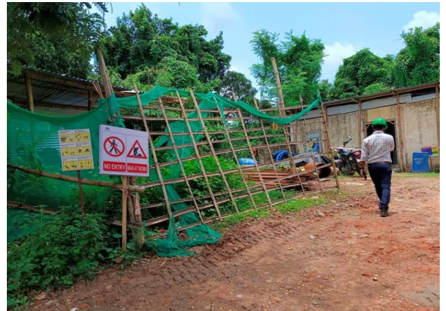
Caution Board placed at site
