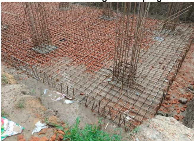
Work progress for Pergola at front garden
