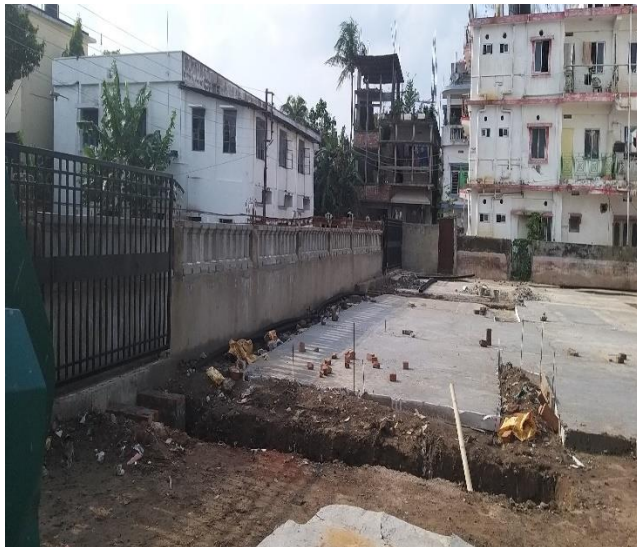
Construction is going on at parking area near Palace
