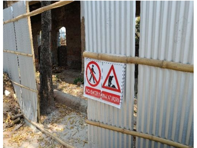
GI sheet – hard barricading at Astabal Area
