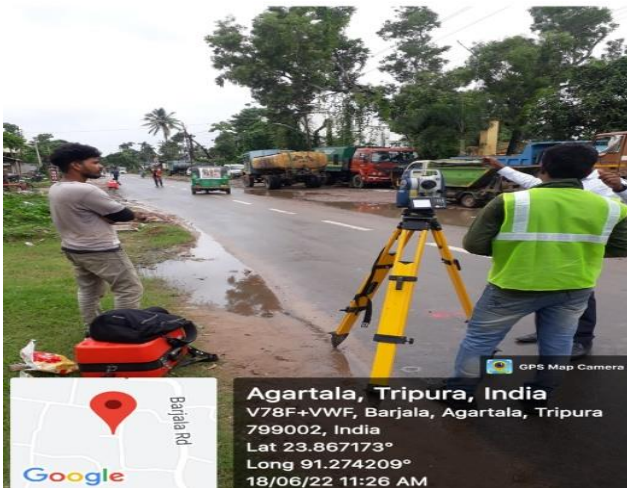
Survey work continued for project Road
