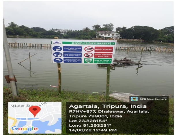
Temporary COVID 19 Information Board at MBB College Lake work site
