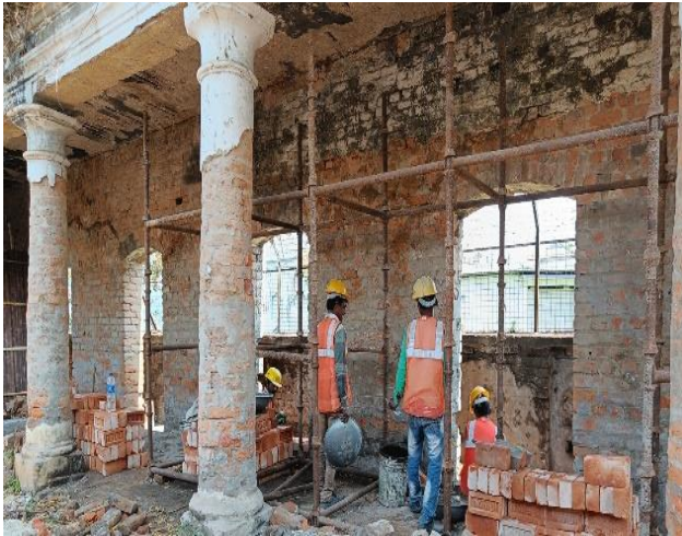
Work continued at Astabal Area. Use of PPEs noted
