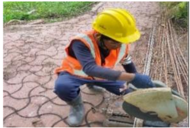
Use of hand gloves during cutting of steel rod at Ujjayanta Palace
