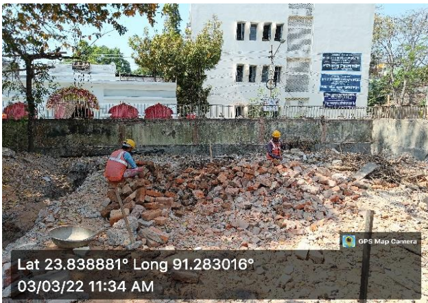
Food Court Demolition work continued
