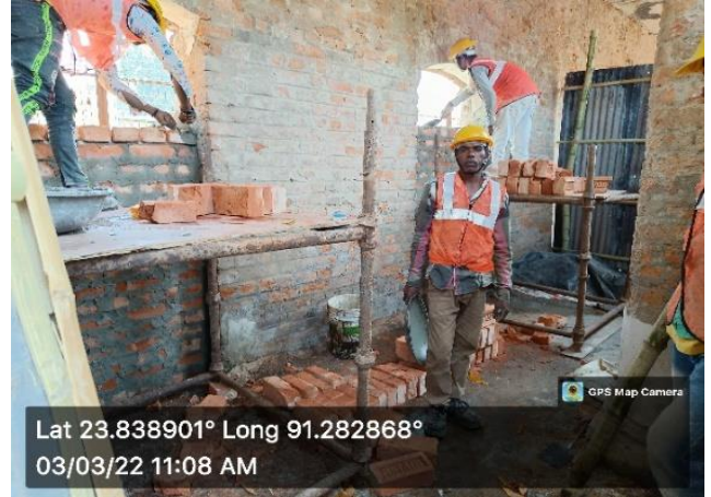
Work started at Astabal Area
